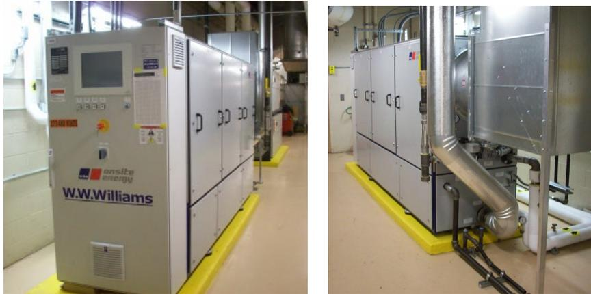
**Figure 6a.** CHP Unit (front and back views with heat recovery piping)
